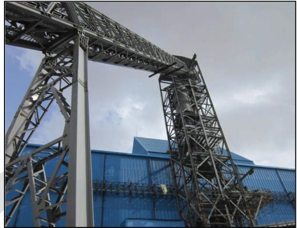
65m tall intermediate DRI silo structures
