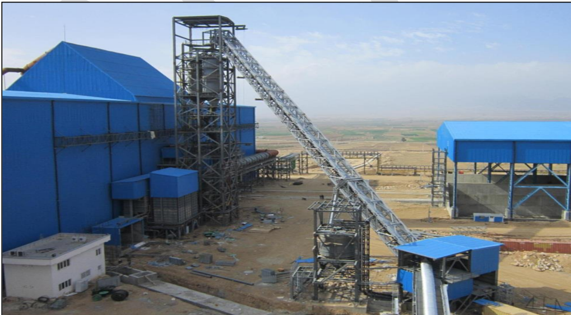
Direct reduced iron transfer sidewall belt implementation- Pasargad Steel (iron smelting) Co.
