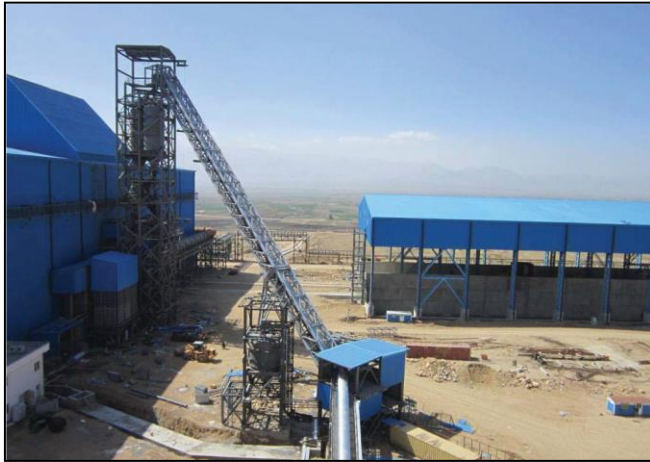
65m tall intermediate DRI silo structures
