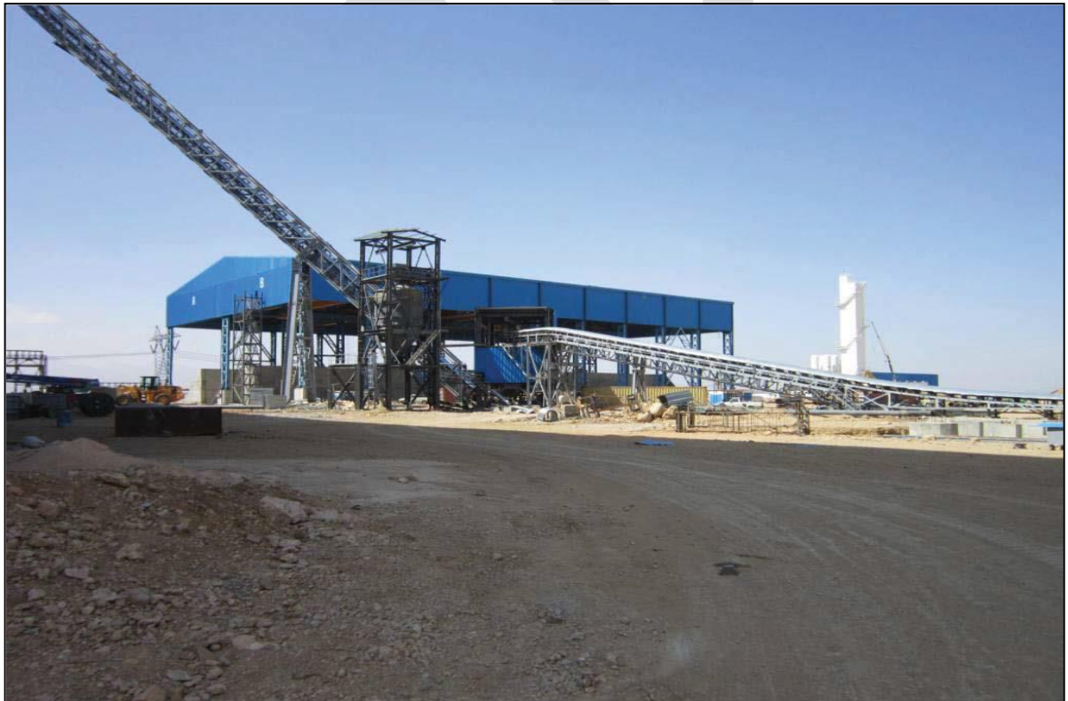
Screen and belts preceding and succeeding DRI silo structures
