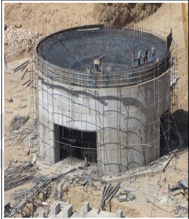
12000 Ton sponge iron storage tank foundation
