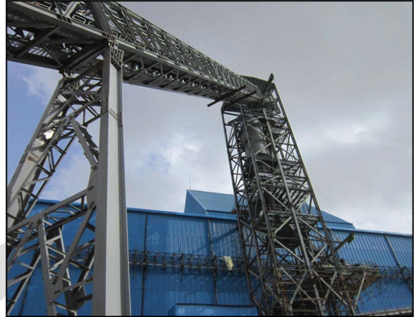
65m tall intermediate DRI silo structures
